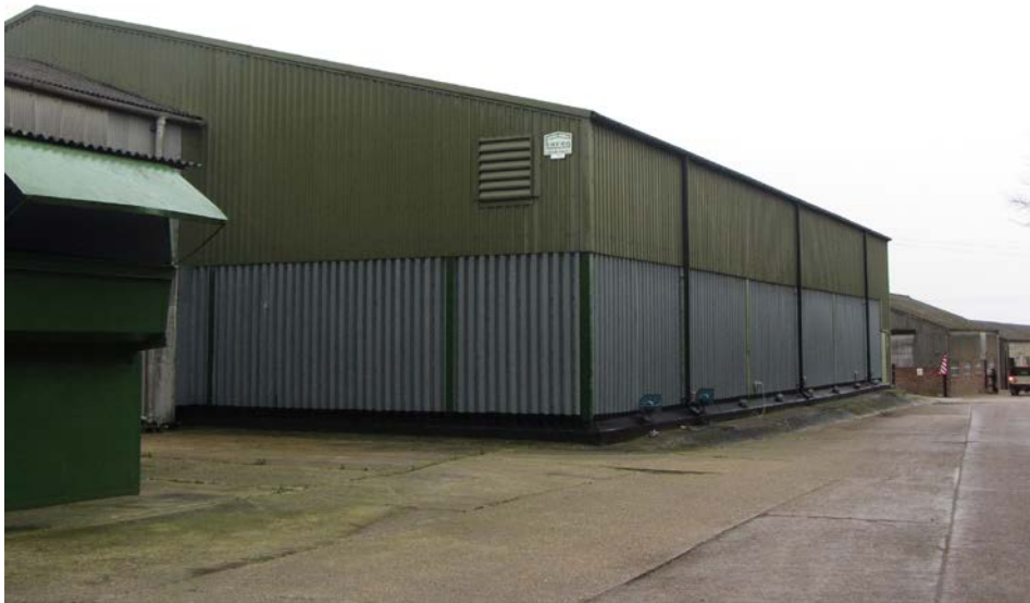
Figure 1 Contemporary barn building with clad in metal sheet
