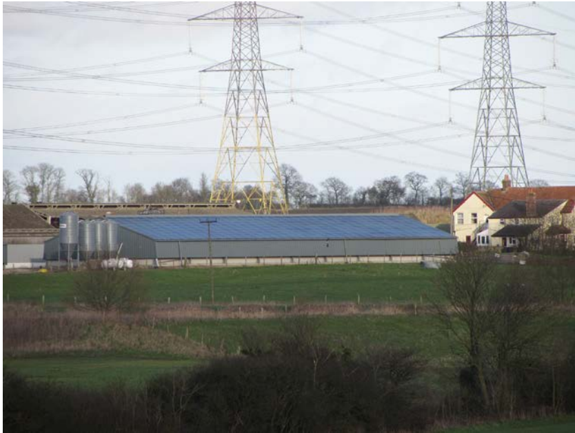
Figure 3 Large scale farm building with solar roof
